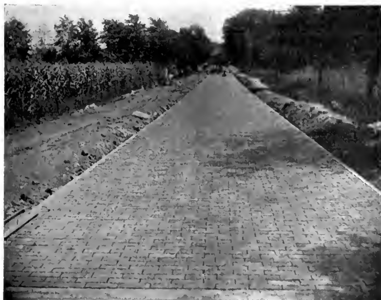
Fig. 2—Completed brick pavement, Paris, Ill.
